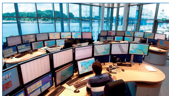
Figure 25 VTS Centre, Travemunde, Germany
