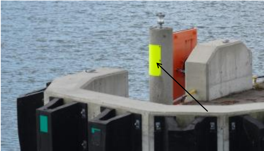
Figure 38 Pier head attached with fluorescent yellow retroreflective material
