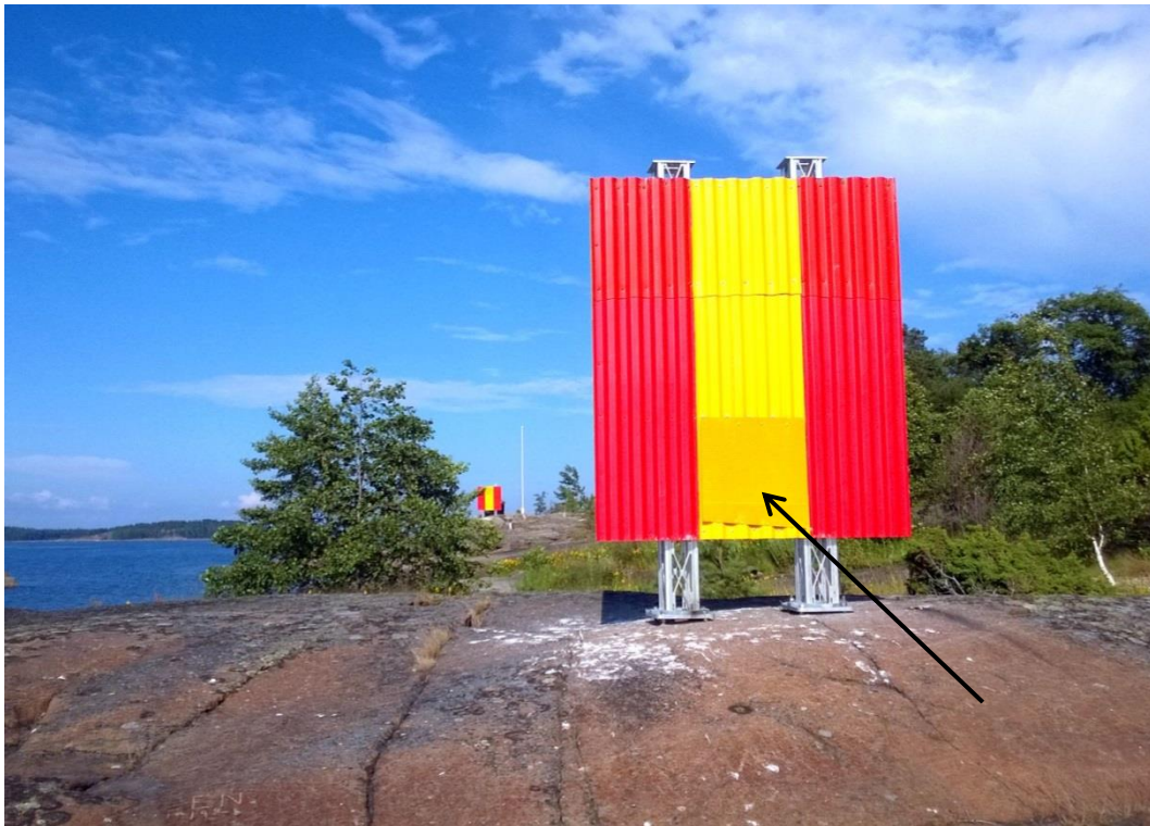
Figure 37 Front day board with partly covering yellow retroreflective sheeting for night time use
