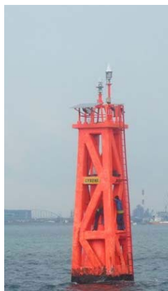
Figure 31 Supporting structure used as a daymark
