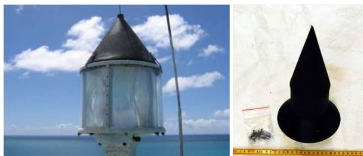
Figure 4 Components designed to reduce landing area
