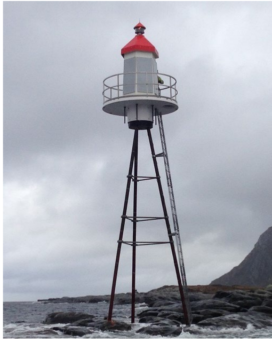
Figure 6 Domberskjera lighthouse with white solar modules
