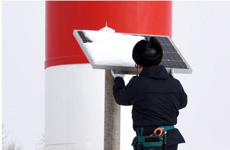
Figure 16 Heavy snow deposits on a solar module in China
