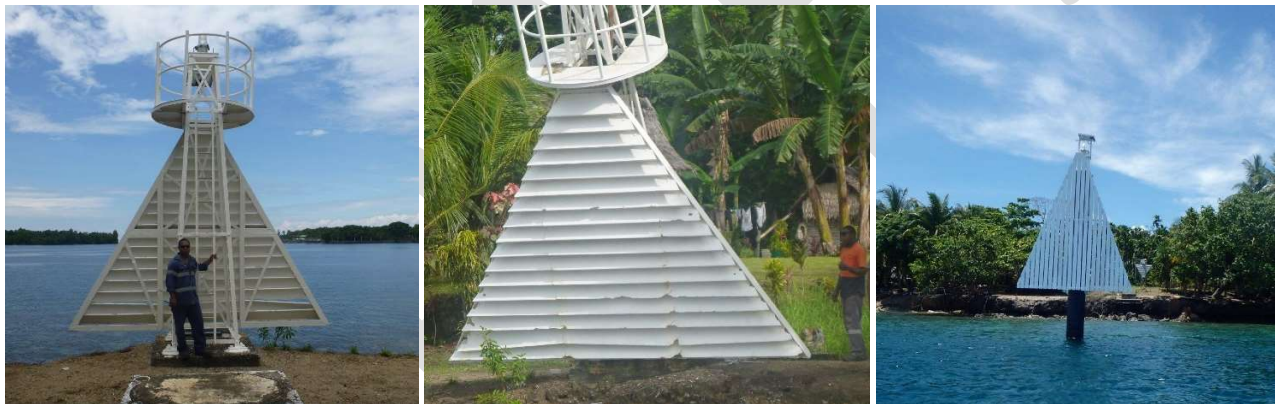
Figure 13 Front Lead dayboard and light – (left to right) rear and front view of land sited light and monopile replacement
