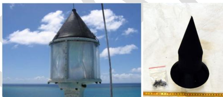
Figure 4 Components designed to reduce landing area
